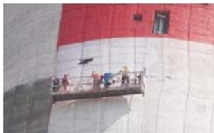
platform are common sites to avoid the accidents. Fall arrestors are also used as an additional protection. People do use wind speed monitors at high altitude work for fixing the schedule.
